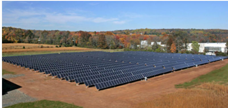
Johnson & Johnson Consumer Companies Solar Farm, Skillman, N.J. Once complete, the SAS solar farm will resemble this structure.
